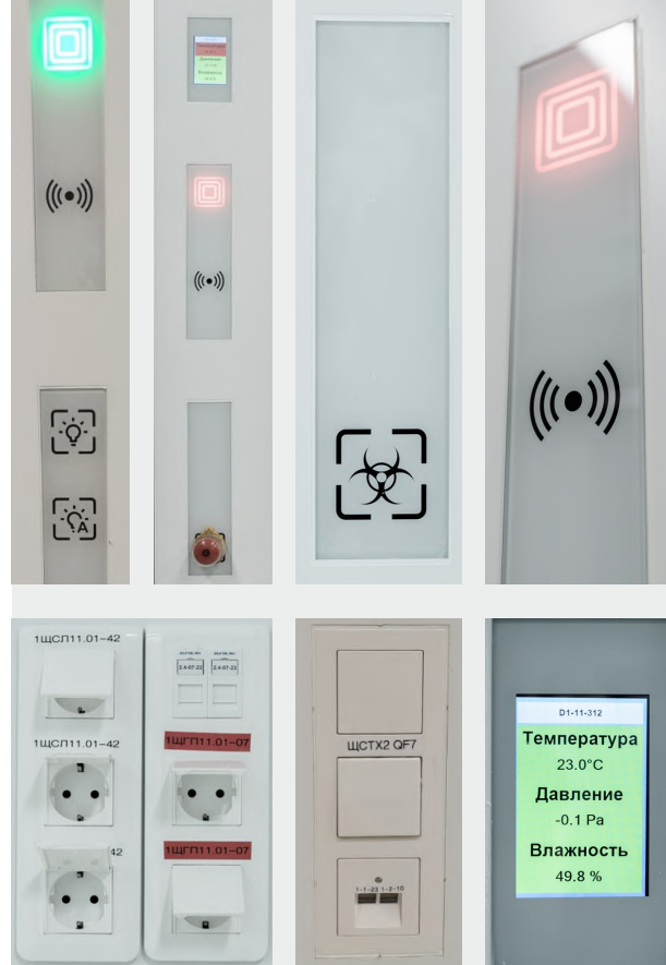
Elements installed in media panels
