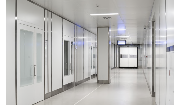
The metal column of the building in the corridor is covered with panels
