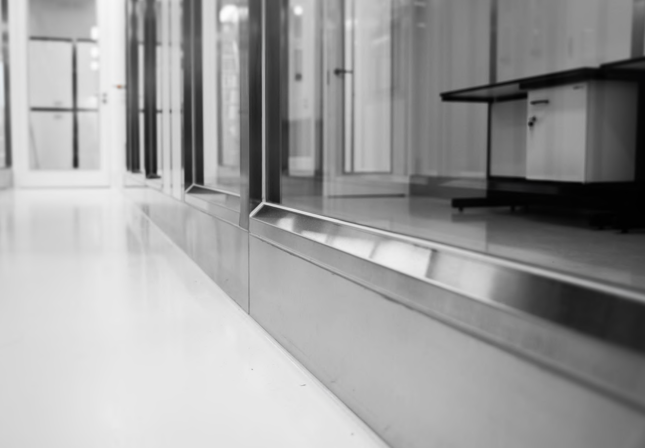
Glass partition, wall post and floor baseboard
