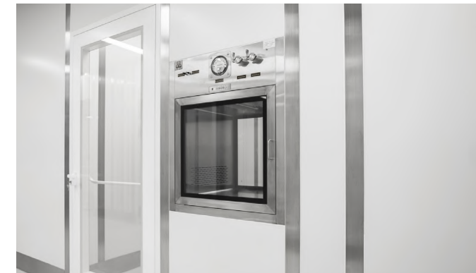
Material airlock. All engineering nets above and below are covered with wall panels
