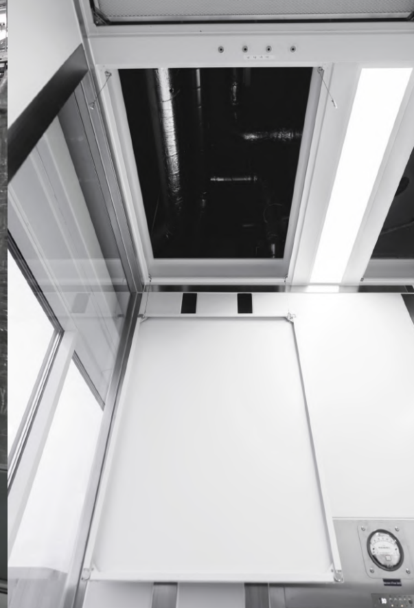
Ceiling panel-hatch for maintenance
