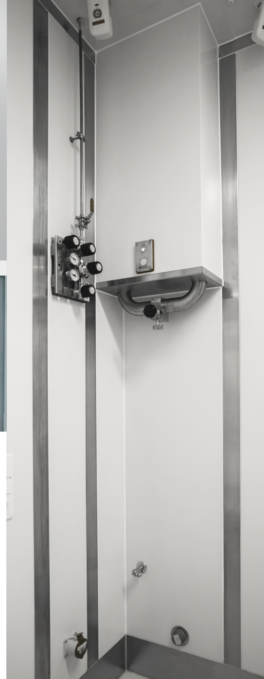
The WFI water loop outlet is covered with wall panels
